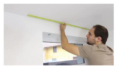
**Example of measurement:** The measured width of the window jamb from the left side to the right is 850 mm, add +200 mm to the parameter (recommendation for installation above the jamb). **Width = 1,050 mm**. You enter the value in bold to the order form.
