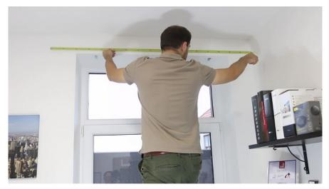
**Example of measurement:** The measured width of the window JAMB from the left side to the right is 1,125 mm, add +200 mm to the parameter (recommendation for installation above the jamb). **Width = 1.325 mm**. You enter the value in bold to the order form.
