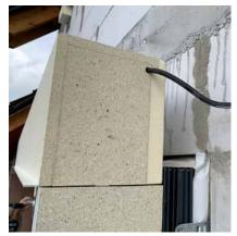
c) Installation in a fully or partially prepared wall pocket
