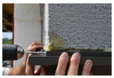
b) Box insertion and levelling
