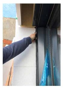
c) Install the jamb using a foam glue (e.g., STY-RO PRO TYTAN). Apply the glue to the edges of the jamb (creating a "frame"). Attention should be paid to installing the jamb vertically aligned (verify either by spirit-level, or by measuring the same area of the remaining visible window frame).
