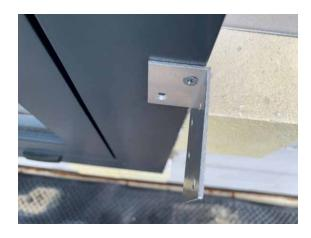
c) Place the jamb to the window frame so that it fits against the angles and anchor it by screws. Anchor the jamb socket inside the box and the jamb through the angles.
