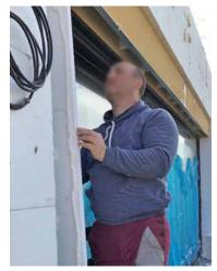
d) It is advisable to secure the jamb in its upper part by a screw driven through the guide rail socket to the box side (the socket must be pre-drilled).
